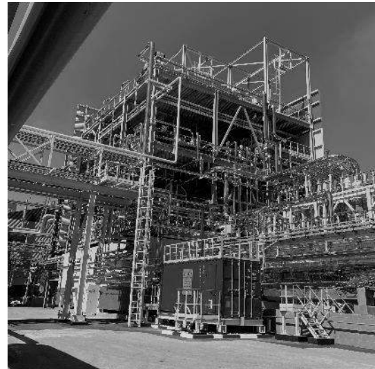
COMMISSIONING OF A 32.5 % UREA SOLUTION PRODUCTION UNIT, 2015 UNIT CAPACITY - 1 200 MTPD
